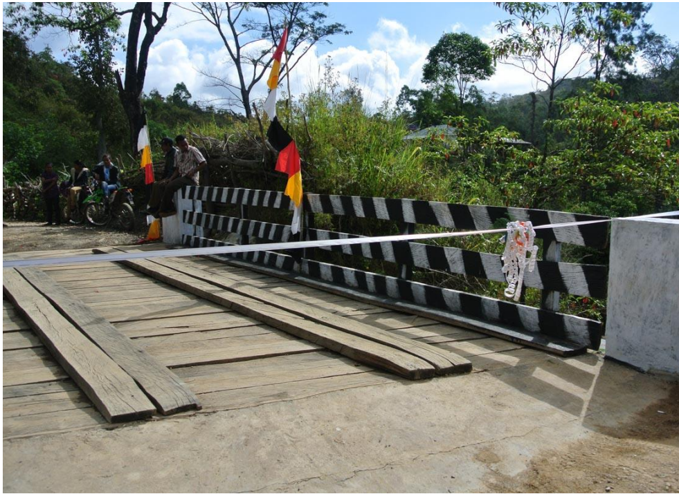
PONTE FOUN IHA ALDEIA HOHOLAU, AILEU
