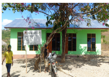
Rehabilitation of health center in village Uma caduak, Laklo/ Manatutu
